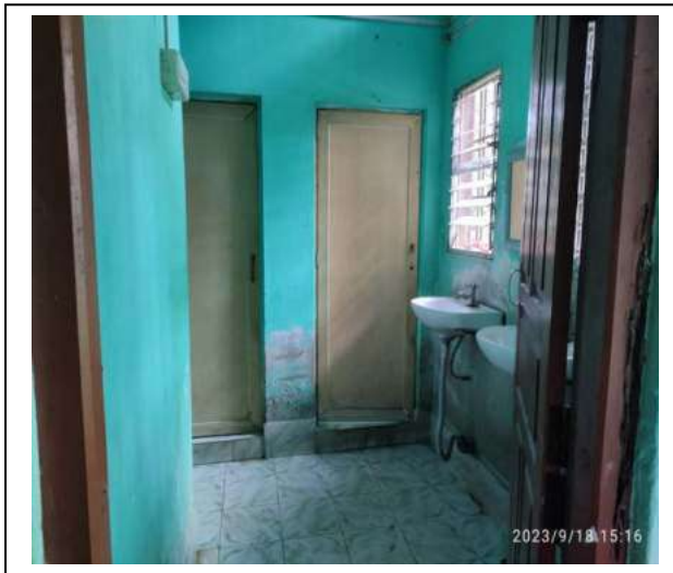
WASHROOM AT GIRLS HOSTEL
