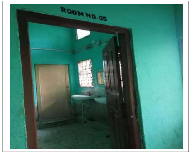
WASHROOM AT GIRLS HOSTEL
